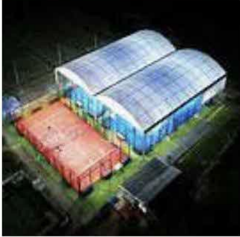
Image screenshotted from page 18 – Precedents, Supporting Background Information from Leonard design architects
