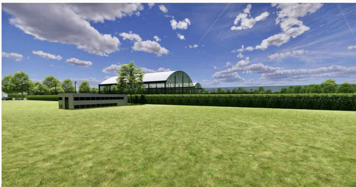
East Glos Club Padel Courts
