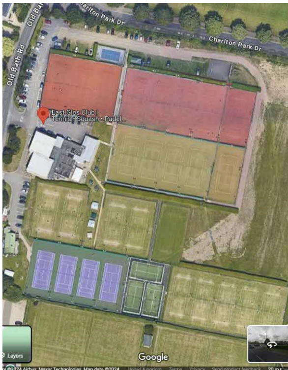
Google aerial images of the East Gos Club in 2024, showing lasting damage to green spaces from previous construction work
